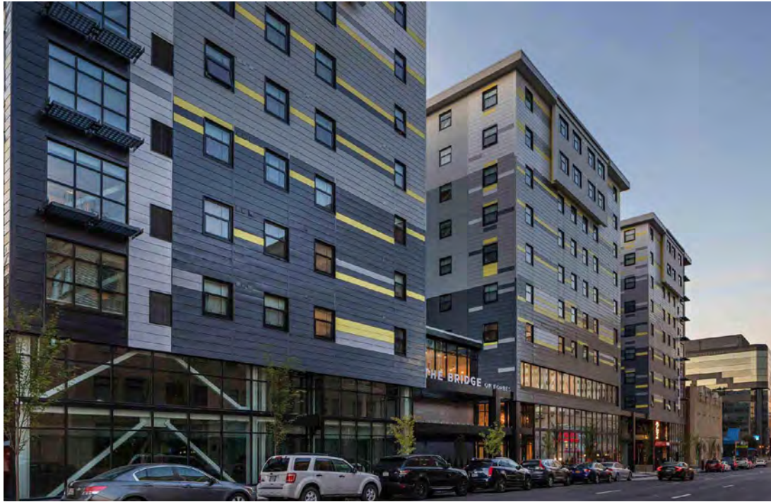
The Bridge of Forbes
