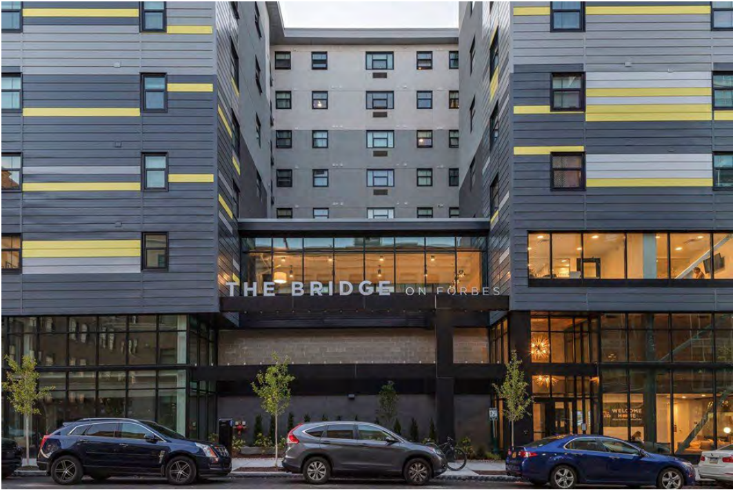
The Bridge of Forbes
