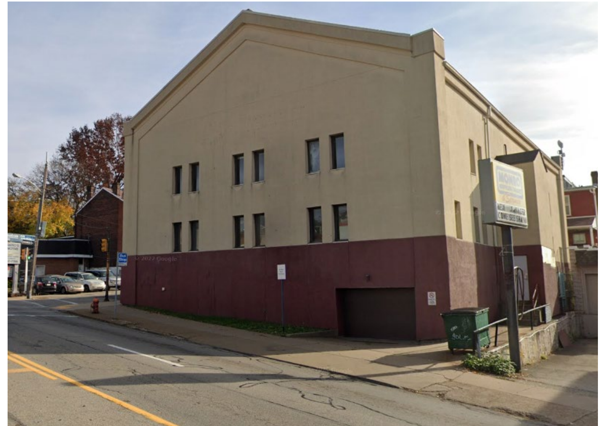
Looking Southeasterly Along Boulevard of the Allies
