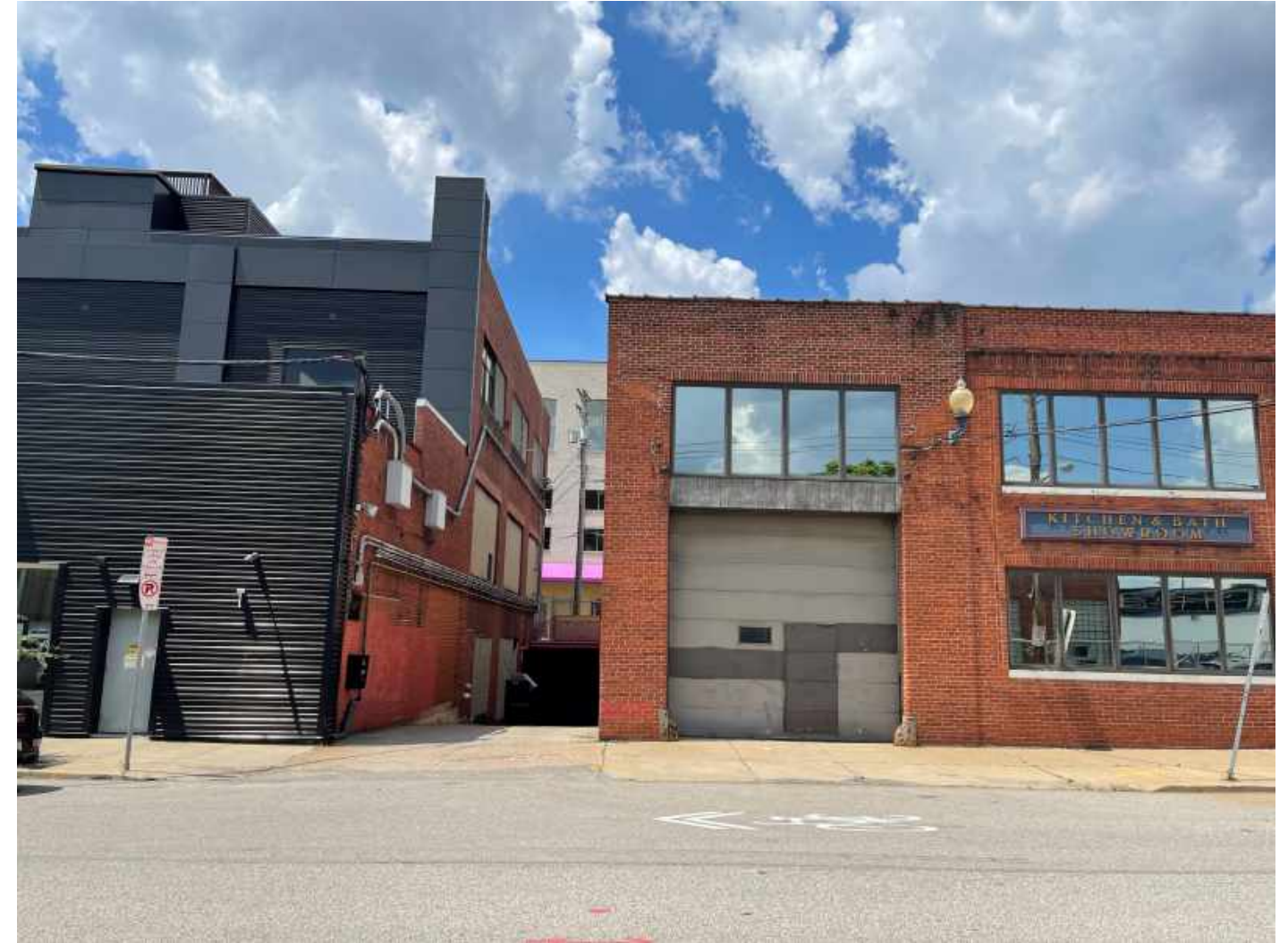
Existing Building Photo – Into Porsche Pittsburgh Drive
