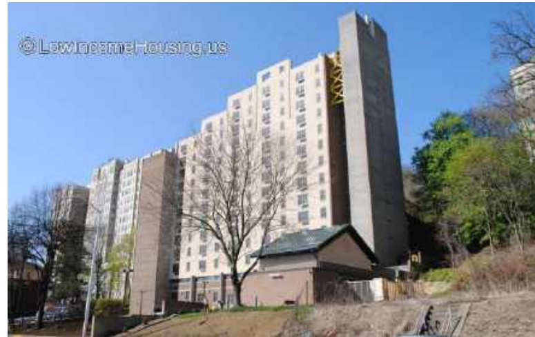
Moorhead Tower 130 ft
