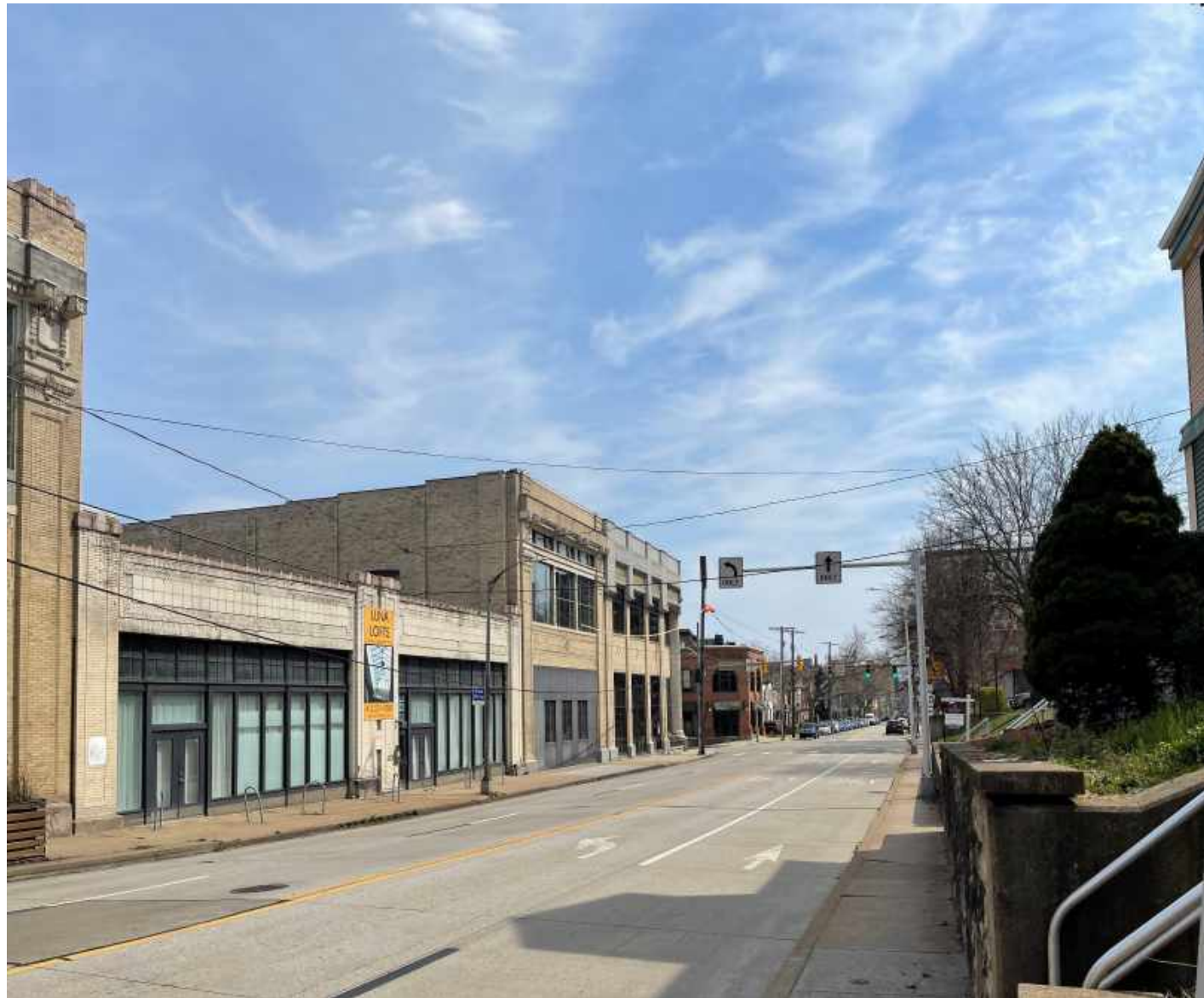
1 View toward Craig Street South, Existing NTS
