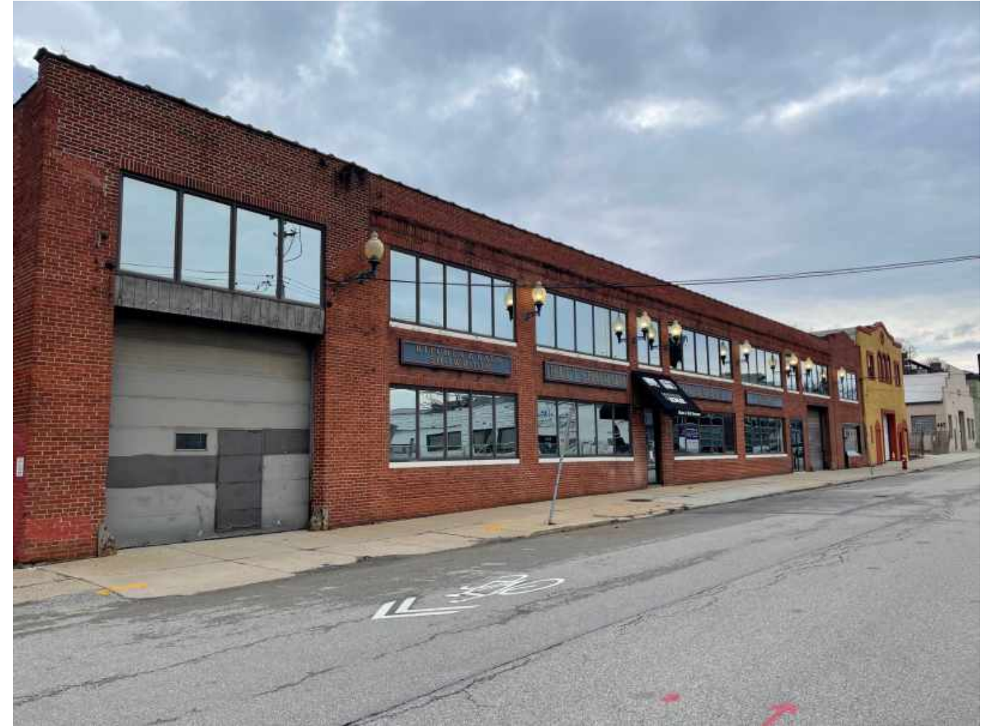
Existing Building Photo – Front Façade along Melwood Avenue
