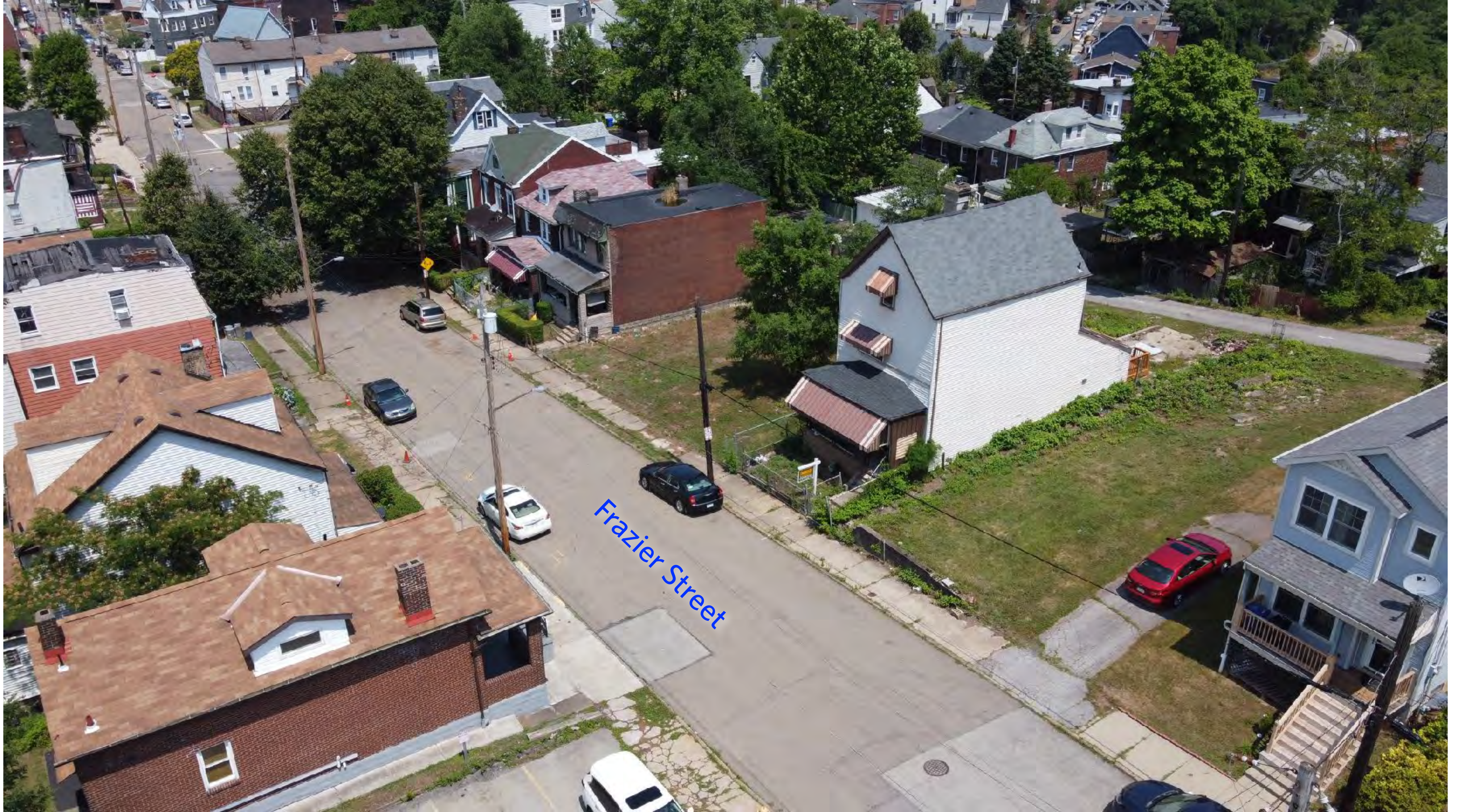
Frazier Street North Infill Residences
