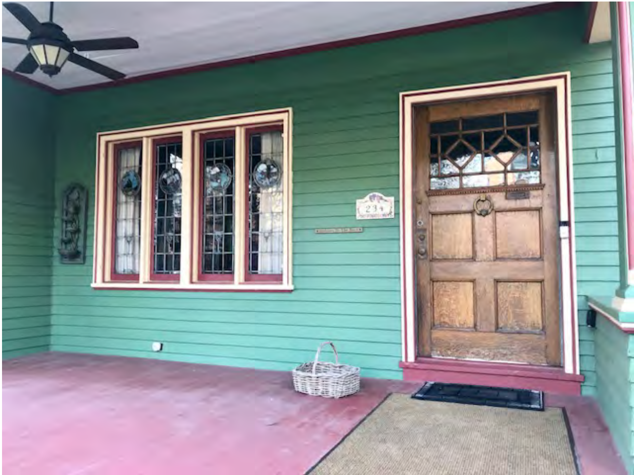
Photo 8. Gallagher-Kieffer House, Front Door and Foyer Windows (Exterior) , March 2020. Source: Matthew W.C. Falcone.
