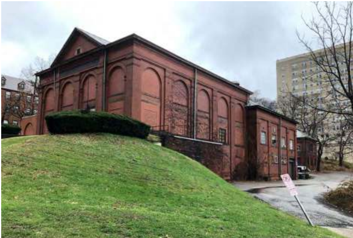
Figure 7. The Pumping Station Building consists of the Pump House facing Centre Avenue (left) and the Boiler House attached behind it. Further to the rear is the detached Laboratory Building.
