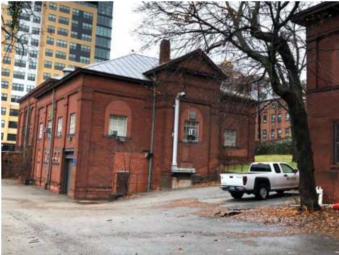
Figure 14. Rear facade of the Pumping Station Building, showing a the projecting center bay on the rear of the Boiler House.
