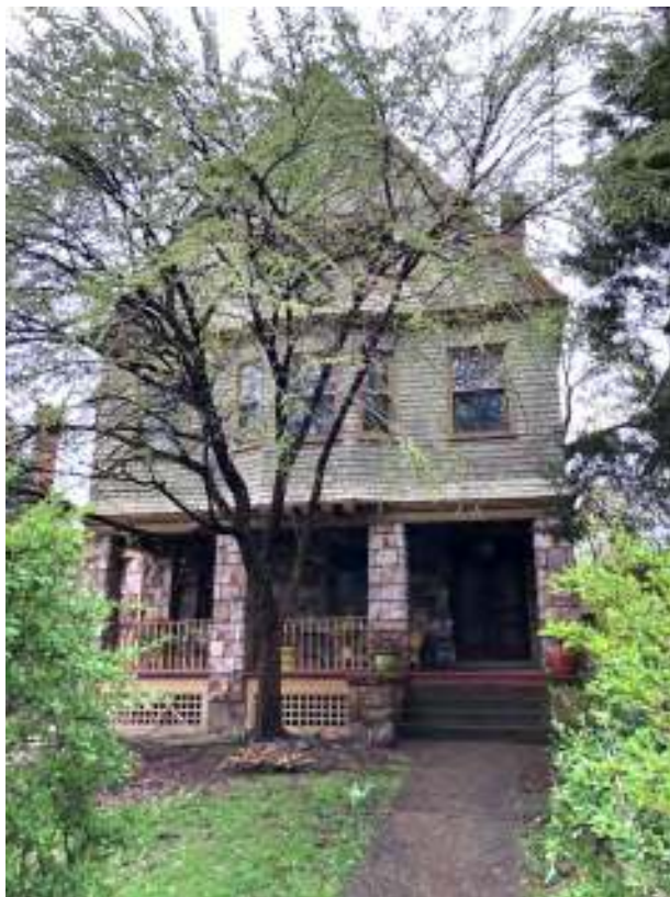
Figure 118. The front elevation of Fraser's house, looking north.
