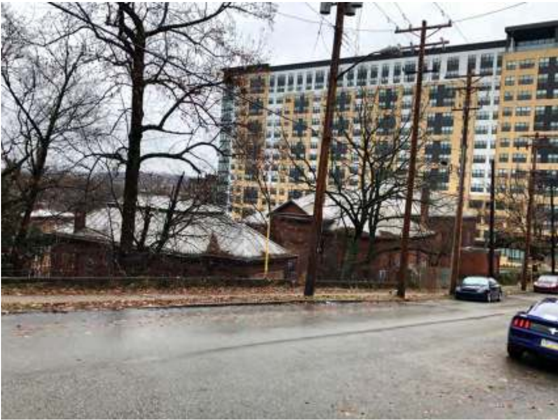
Figure 4. Looking down N. Dithridge Street to the south, showing (from left to right) the Laboratory Building, the Pumping Station Building, and One on Centre.
