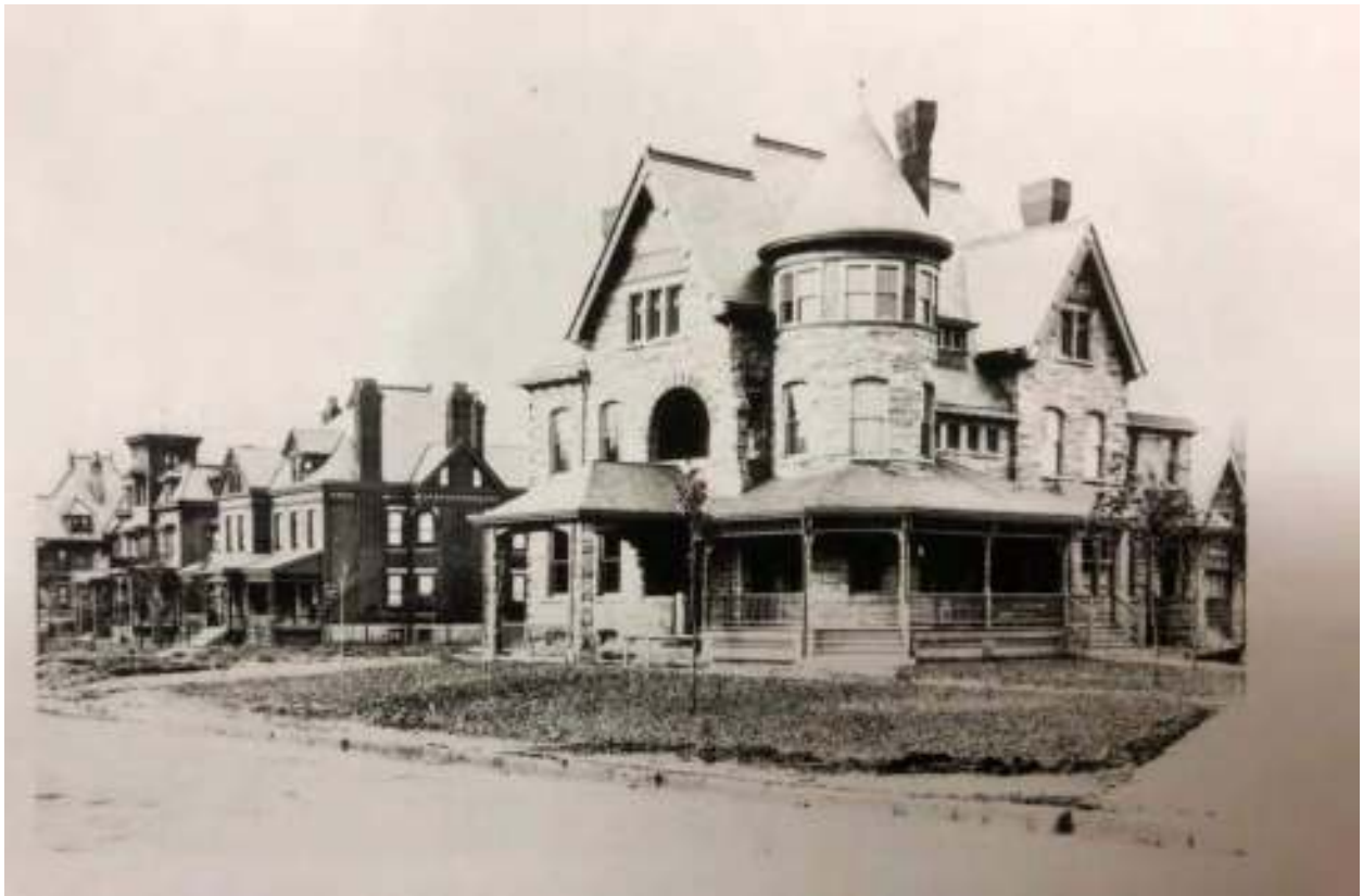
Figure 89. The Dr. Thomas A. Rex House on the corner of Ellsworth Avenue and Neville Street. The image was taken sometime between late 1888 when the house was completed and 1898, when the Church of the Ascension was constructed in the empty lot to the north of the house (Carnegie Library of Pittsburgh).
