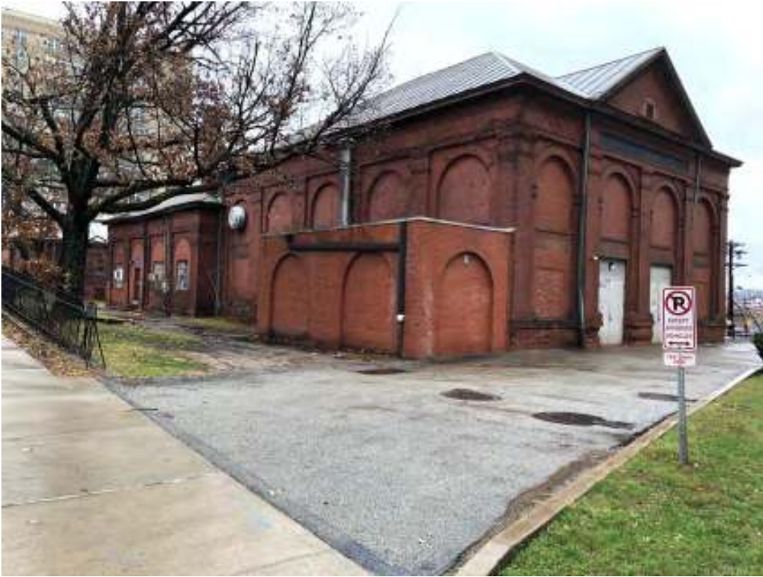
Figure 10. The Pump House, looking northeast, showing the four-bay wide front facade and five-bay wide west facade with the Boiler House to the rear.
