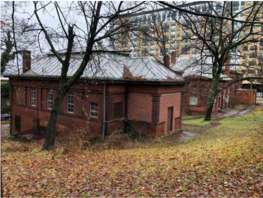
Figure 38. The Laboratory Building, looking southeast, showing the bricked-in entry porch of its front (west) facade.
