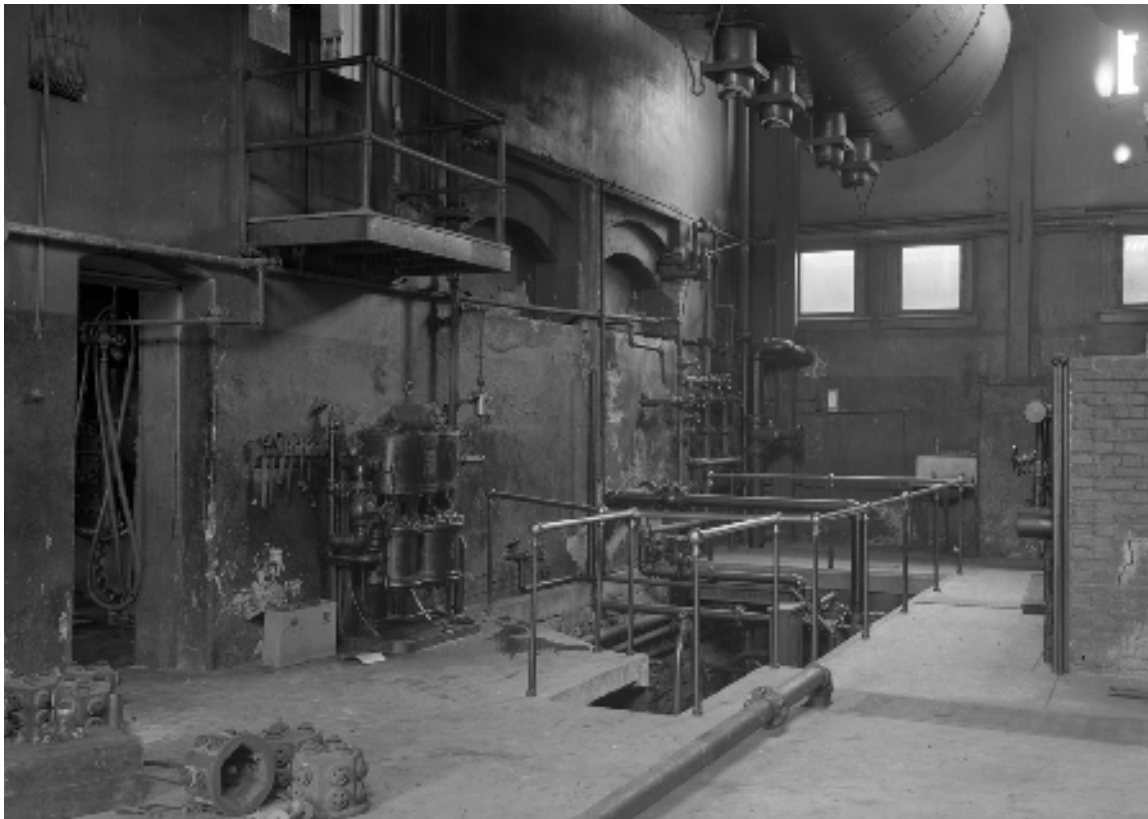
Figure 30. Interior of the Boiler House, December 8, 1915, looking southwest, showing a balcony (top left) that allowed workers in the Pump House to see into the Boiler House (Historic Pittsburgh).
