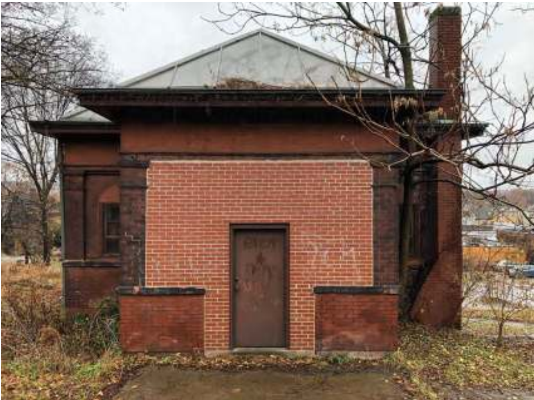
Figure 39. Front facade of the Laboratory Building, looking east.
