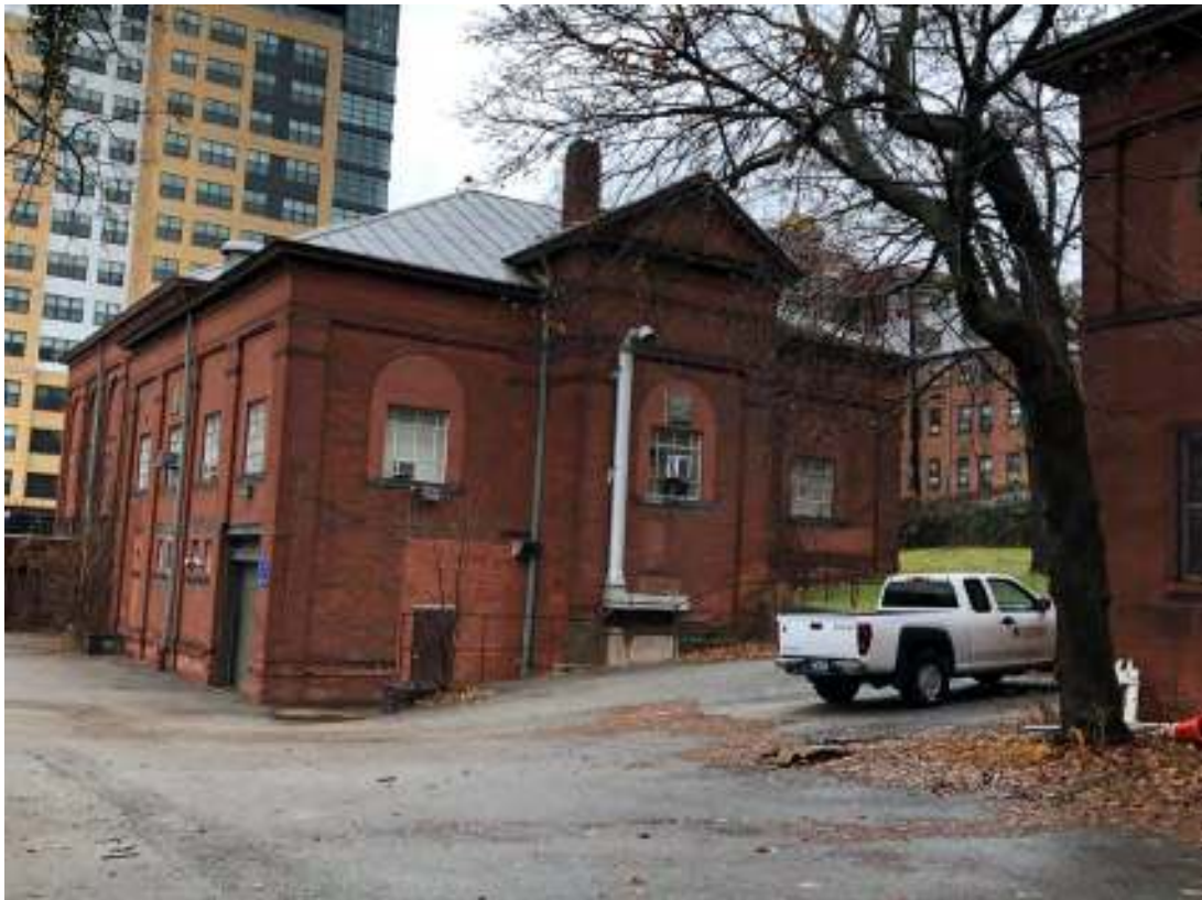
Figure 9. Rear facade of the Pumping Station Building looking south, showing the rear of the Pump House.
