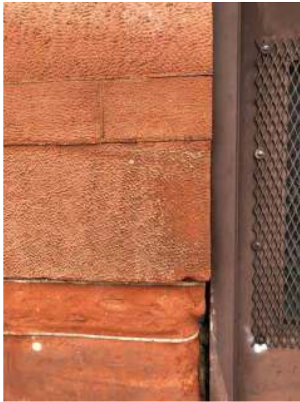
Figure 40. Laboratory Building, showing typical foundation stone details.
