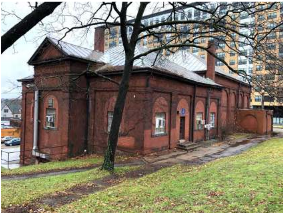
Figure 15. Rear and west facades of the Pumping Station Building, looking southeast.
