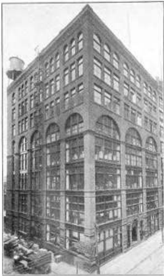
Figure 113. 1908 photograph of the Arbutnot-Stephenson Building, showing Fraser's modern use of vast expanses of glass on the lower stories ( The Story of Pittsburgh and Vicinity: Illustrated , Pittsburgh Gazette Times, 1908).
