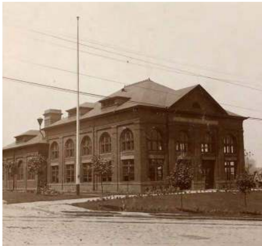
Figure 17. The Pumping Station Building c. 1900, showing the large corbeled brick chimney (left) that vented exhaust from the coal-fired boilers in the Boiler House (Harry B. Johnston, Carnegie Library of Pittsburgh).
