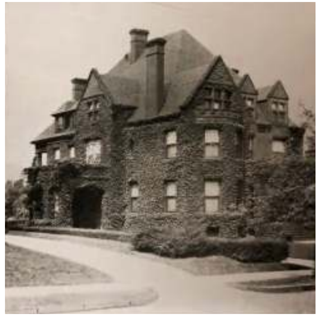
Figure 124. South facade of the H.S.A. Stewart house, c. 1902 (Carnegie Library of Pittsburgh).
