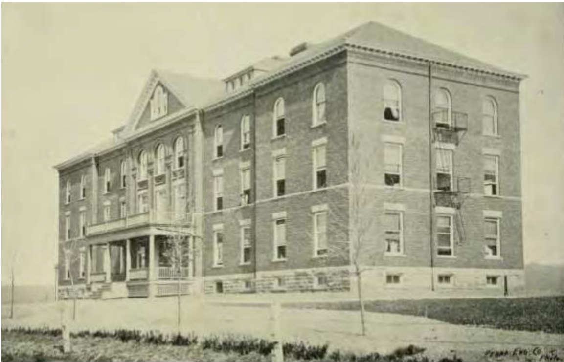
Figure 137. Silas M. Clark Hall, the boys' dormitory designed by Fraser, showing Classical Revival details that he would again employ for the Herron Hill Pumping Station ( Twenty-Ninth Annual Catalogue of the Indian Normal School of Pennsylvania, 1902-03 ).
