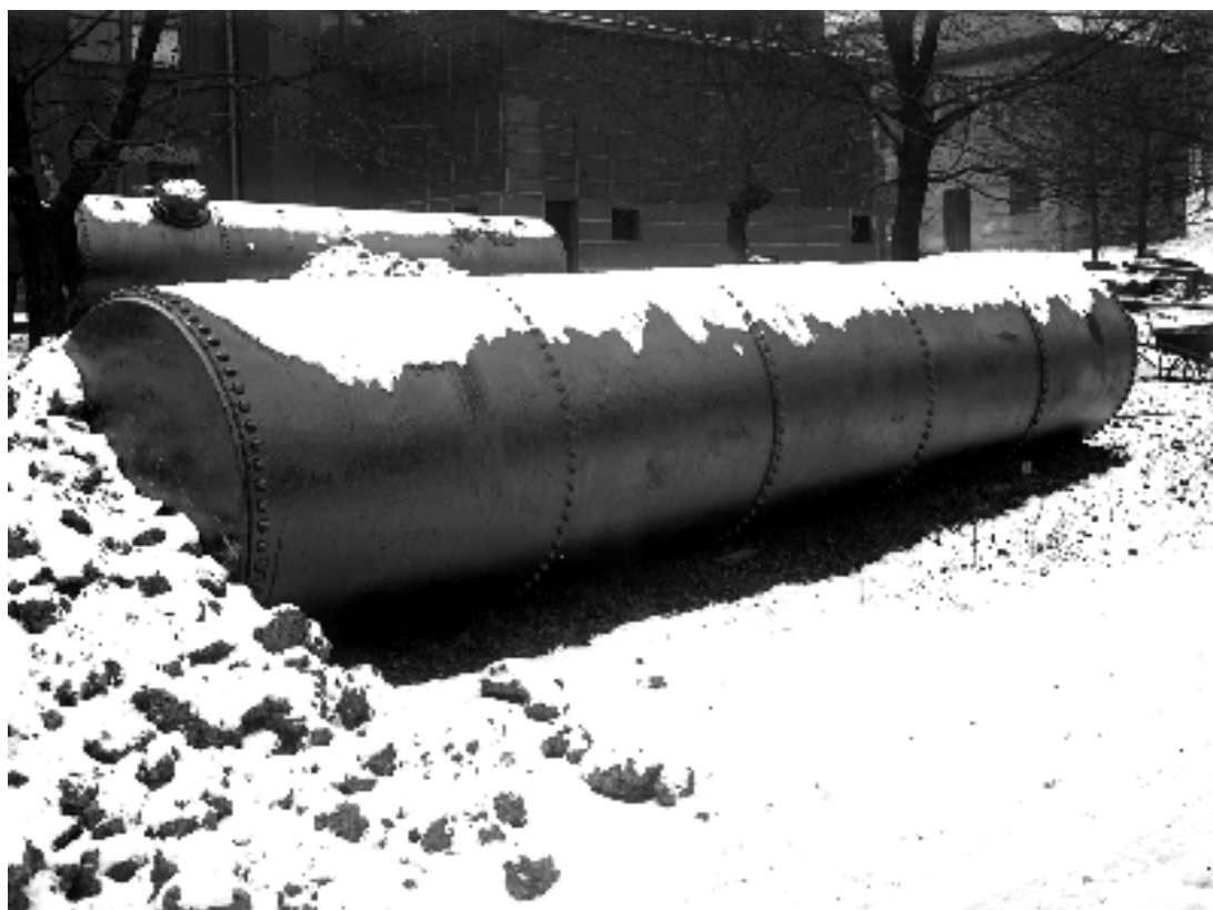
Figure 33. The east side of the Boiler House, January 4, 1919, looking northwest, showing new oil tanks that will soon be buried in the east yard. At the top center is a temporary frame enclosure attached to the east side of the Pump House to facilitate construction (Historic Pittsburgh).
