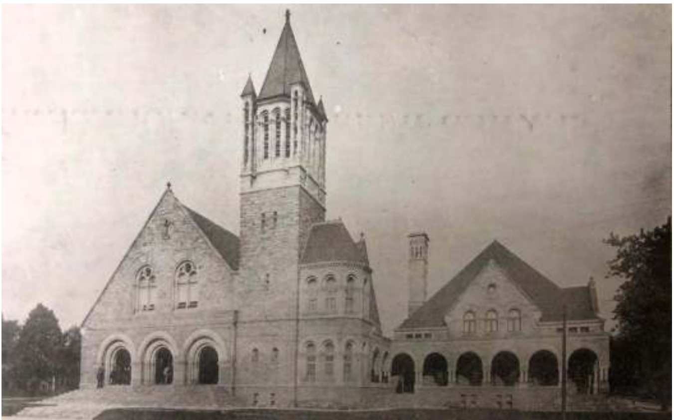
Figure 134. Eastminster United Presbyterian Church in East Liberty, 1896, showing the Church (left) and the attached Sunday School Building (right). At the time, this was Sixth United Presbyterian and Fraser's home church ( Greater Pittsburgh: The "Iron City," Illustrated, 1896, New York: The Graphic, 1896 ).
