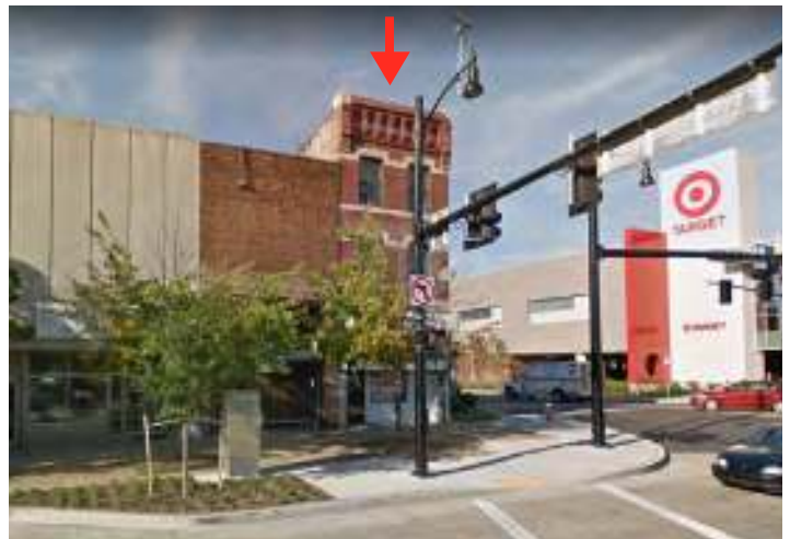
Figure 86A. The Denholm Building shortly before its 2018 demolition (Google Street View).
