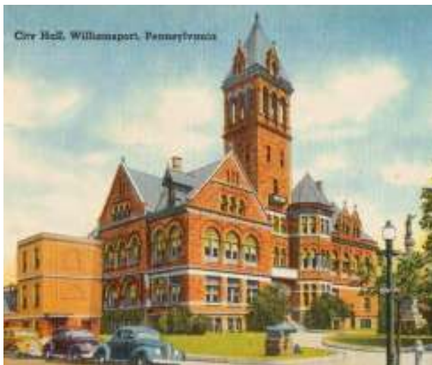
Figure 138. Williamsport City Hall, alleged by Fraser in a lawsuit to be a copy of his design for the Carnegie Library in Allegheny (detail from an undated postcard).
