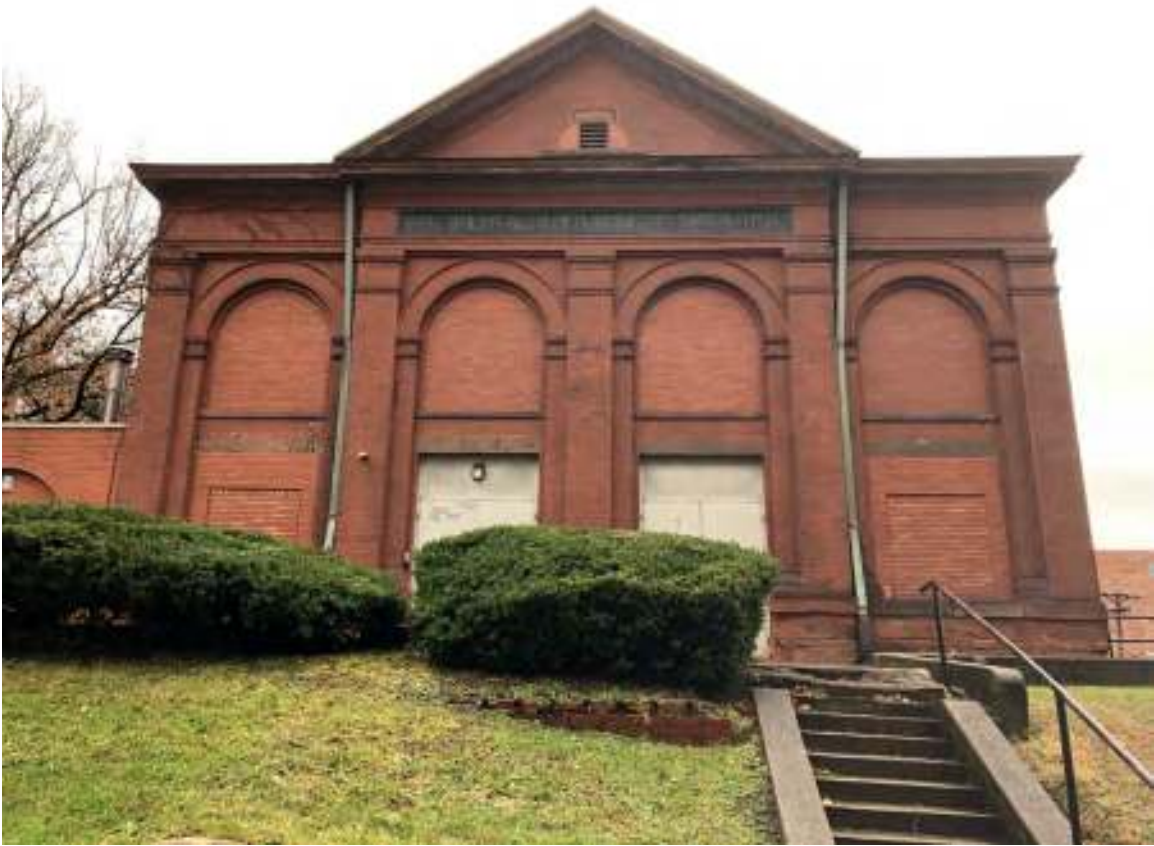
Figure 12. Front (south) facade of the Pumping Station Building, showing the formality and symmetry of William S. Fraser's Classical Revival design.
