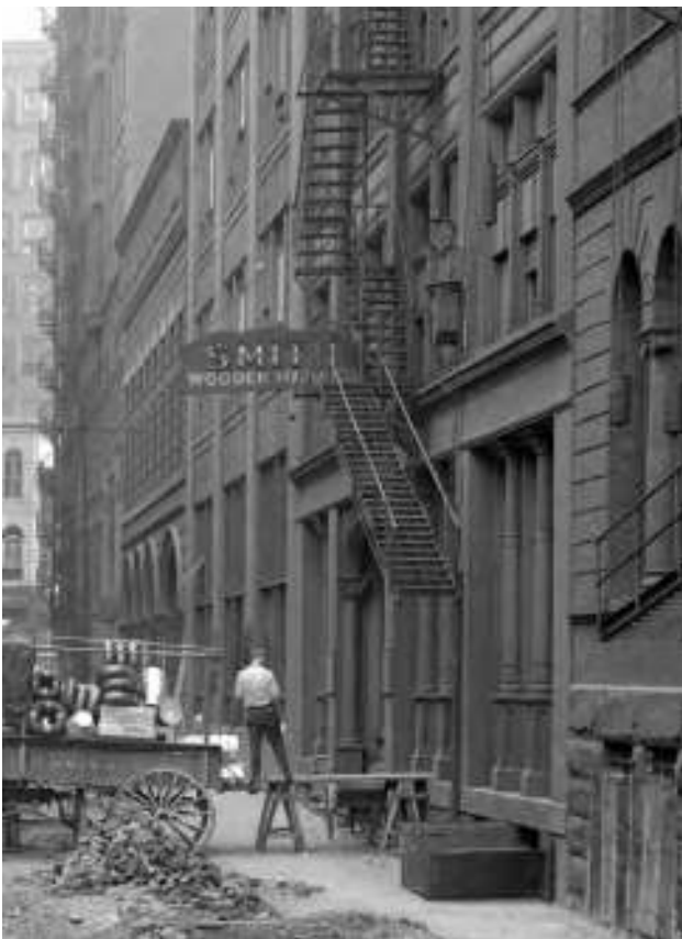
Figure 121. Eighth Street in 1915, looking south toward Penn Avenue, showing the four-bay-wide Smith Woodenware Company. Prior to 1906, the three left bays were home to the Gensenleiter Livery and the right-most bay was the site of the three-story building that housed Fraser's office (Pittsburgh City Photographer Collection, Historic Pittsburgh).
