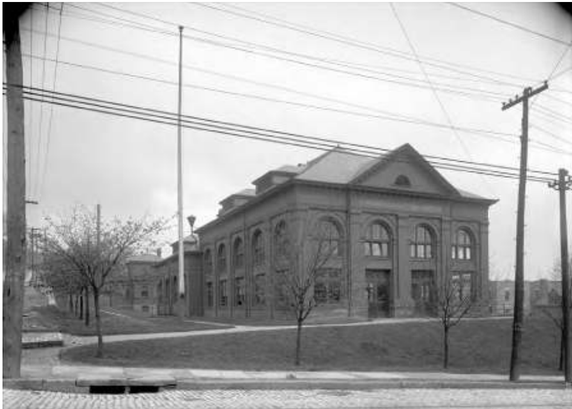
Figure 16. The Herron Hill Pumping Station in 1907, showing original windows and doors, hipped dormers on the roof and a tall flag pole that stood in the west lawn (Historic Pittsburgh).
