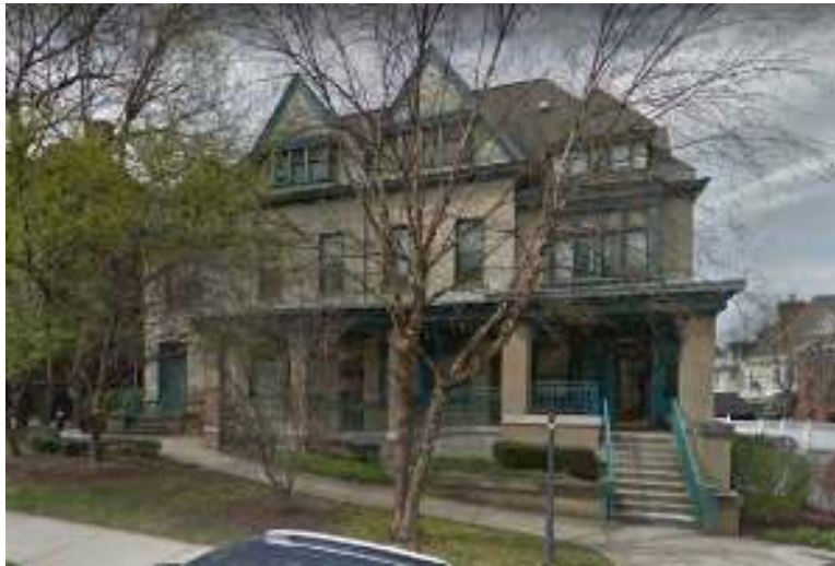
Figure 98. 512 Shady Avenue (Google Street View)
