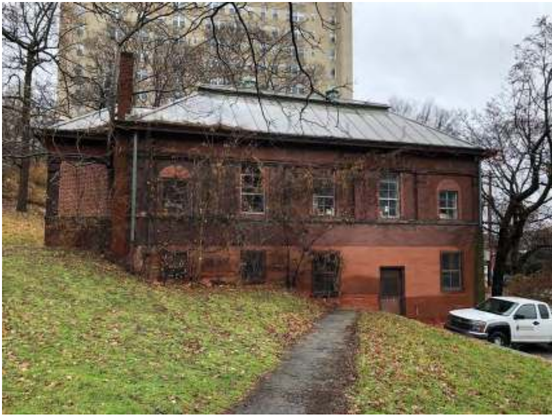
Figure 42. South facade of the Laboratory Building, looking north.
