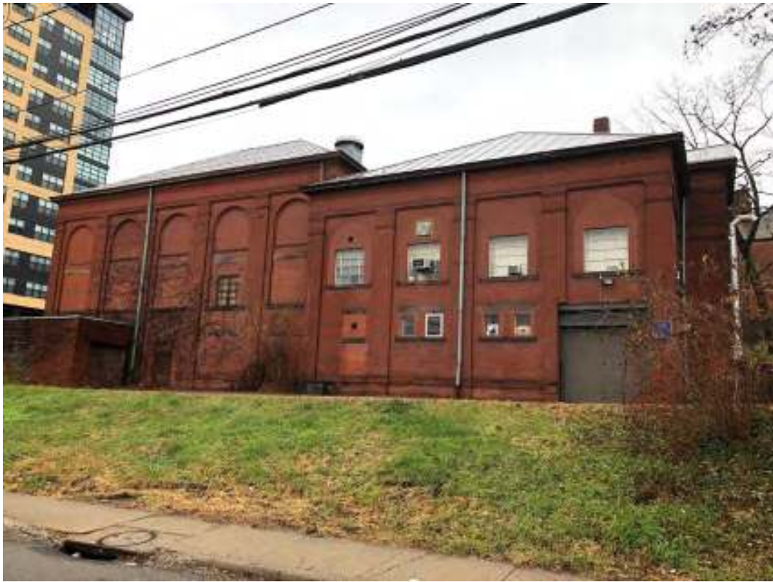
Figure 8. East facade of the Pumping Station Building looking west, showing the lower height of the Boiler House (right).
