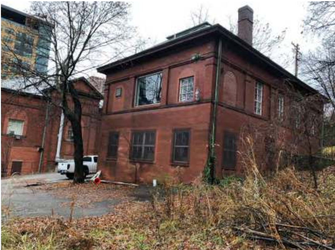
Figure 41. East and north facades of the Laboratory Building, looking southwest.
