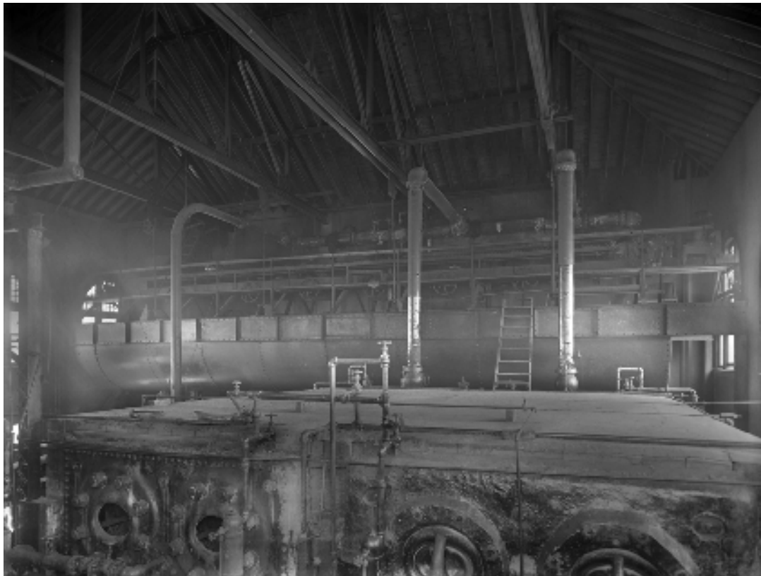
Figure 29. Interior of the Boiler House, October 12, 1912, looking south, showing the open double-height space and steel truss roof system above (Historic Pittsburgh).
