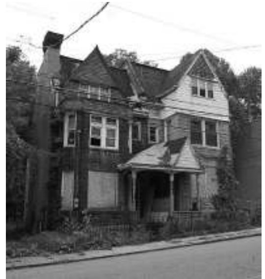
Figure 95. One of a dozen houses to survive into the twenty-first century, shown prior to its rehabilitation (Trek Development).
