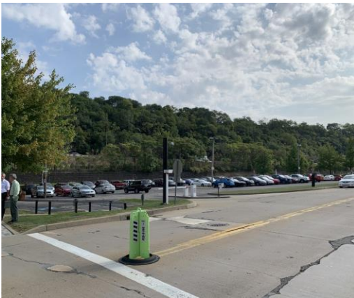
Crosswalk on Technology Drive
