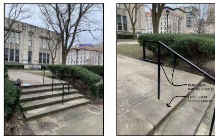
9 PHOTOS - LOCATION #1 - EXISTING
