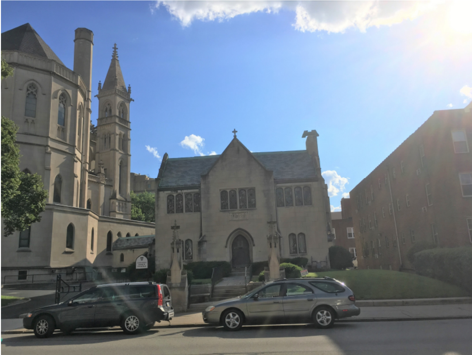
SYNOD HALL, VIEW WEST, DIRECTLY ACROSS N. CRAIG STREET
