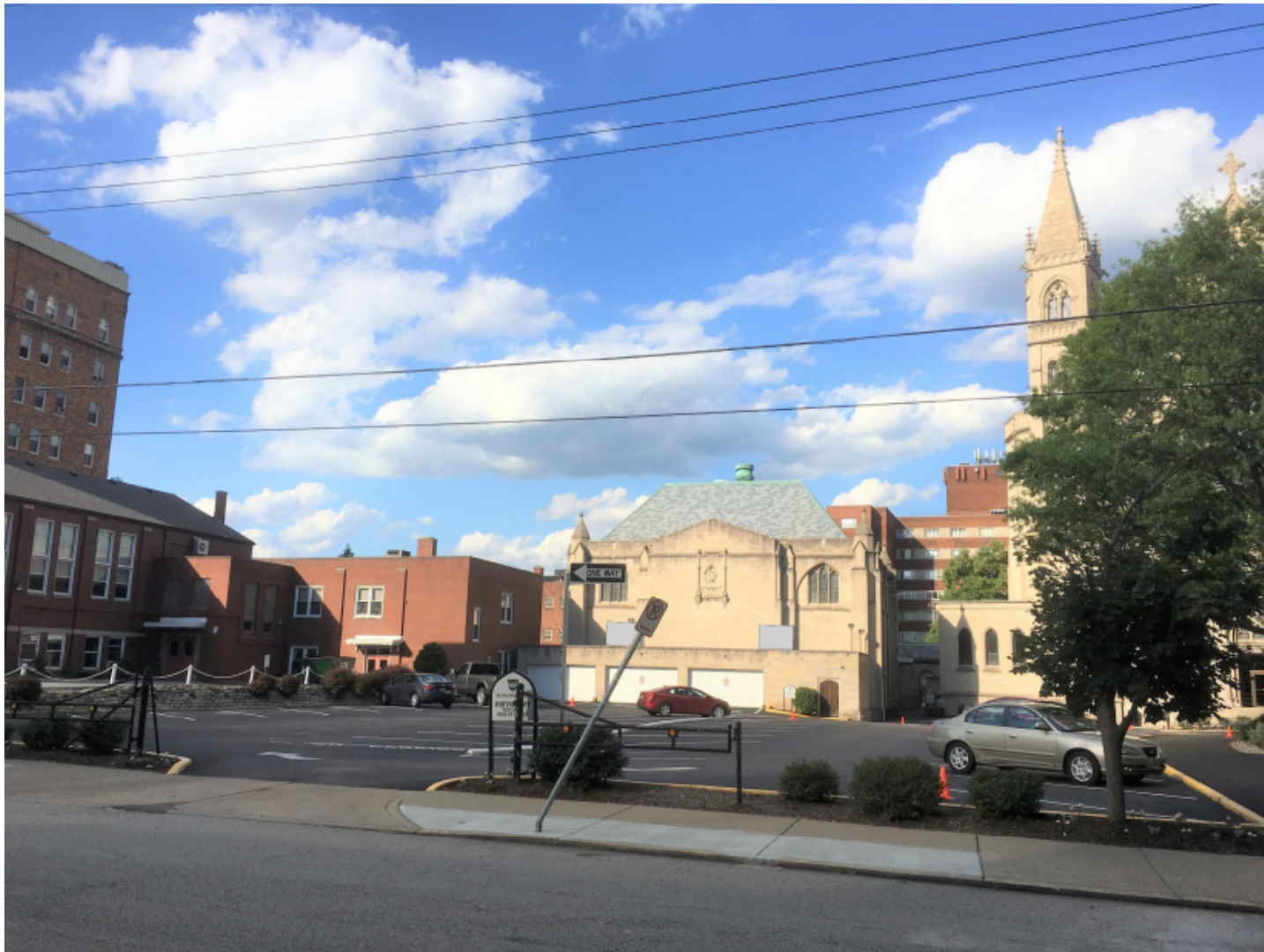
VIEW OF SYNOD HALL FROM ACROSS N. DITHRIDGE STREET WITH PROPOSED ROOFTOP UNITS
