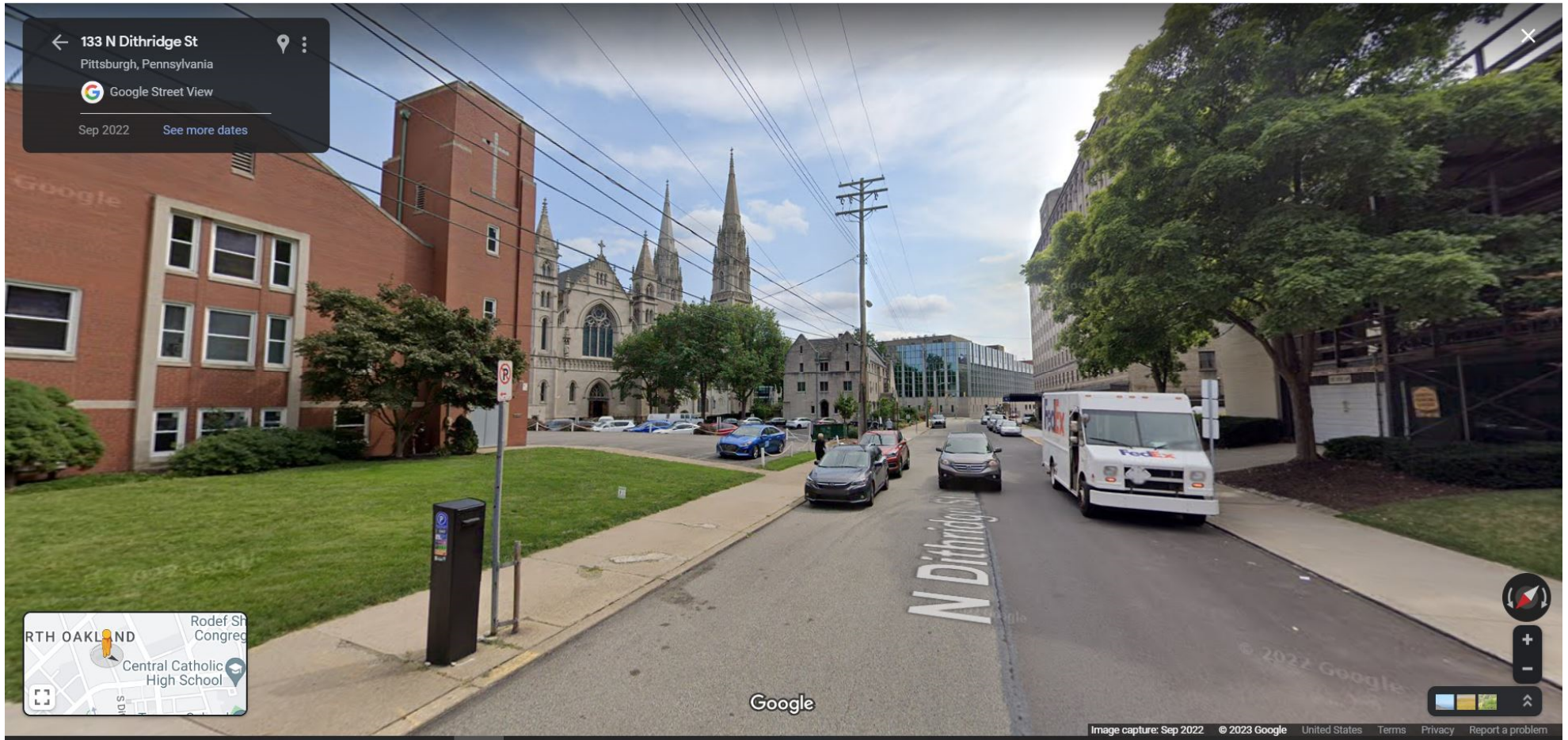
VIEW TOWARD SYNOD HALL FROM N. DITHRIDGE STREET LOOKING SOUTH
